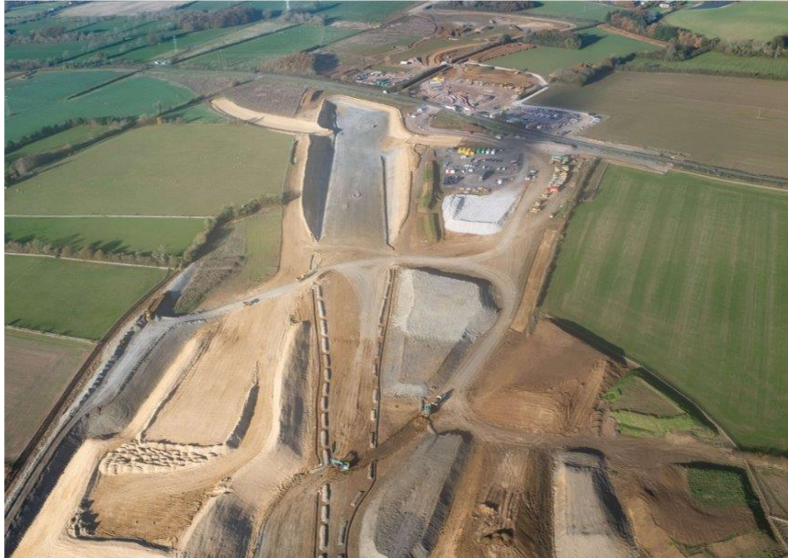
Initial Excavation to Turweston Cutting
