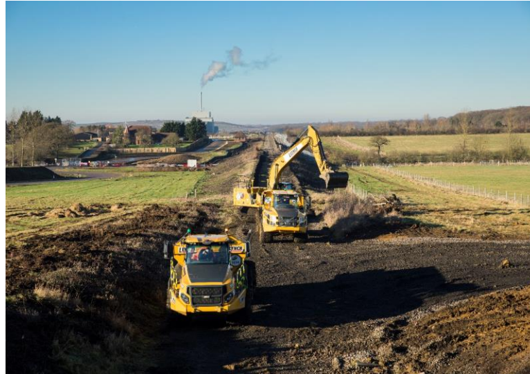
Removal of MCJ line, Grendon Underwood
