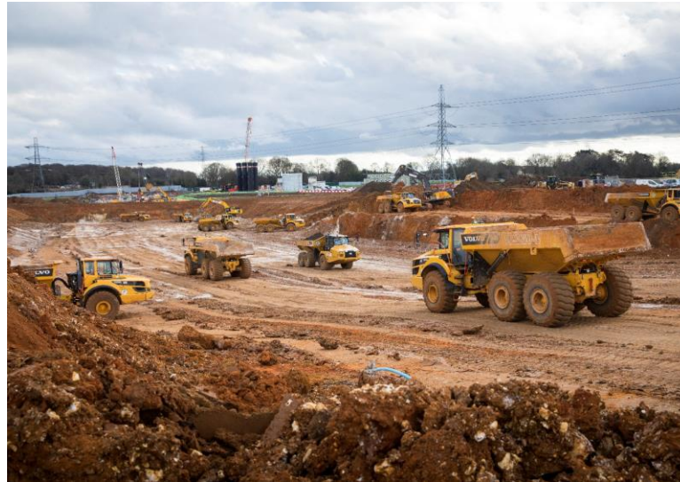
Excavation to South Heath Cutting, Gt Missenden
