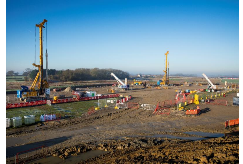
Piling to Perry Hill Overbridge, Twyford
